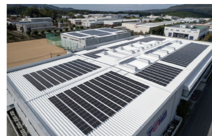
Kyoto East Plant
