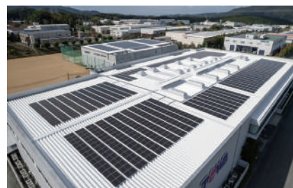
Kyoto East Plant
