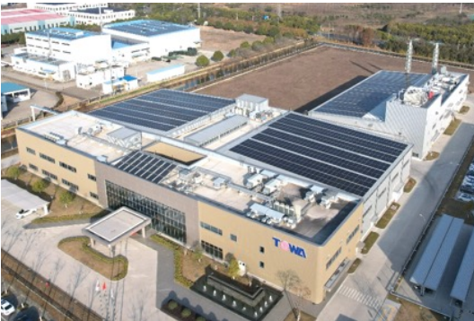
Solar panels installed at the Nantong Plant
