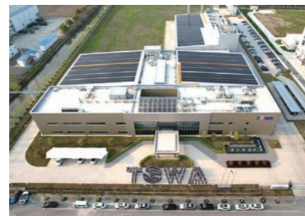
Solar panels installed at the Nantong Plant
